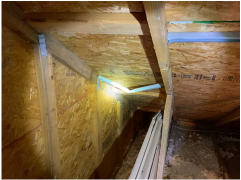
Bent truss stabilizers
