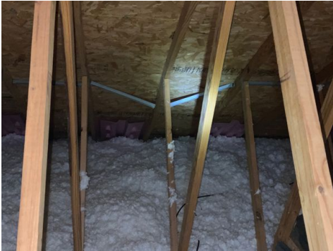
Bent truss stabilizers
