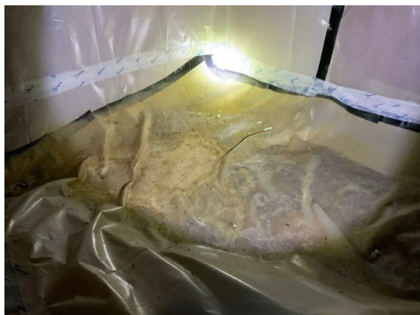
Crawlspace floor was soft indicating moisture intrusion.
