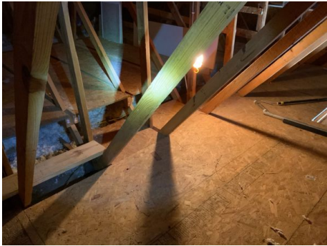
Trusses had been modified for storage. Recommend evaluation by a qualified professional.
